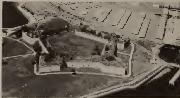
HISTORIC FORT INDEPENDENCE at Castle Island, South Boston, is scheduled in 1976 for a major restoration project. The adjoining area contains a harbor-side park, walkway, picnic tables, Pleasure Bay's sailing pavilion and beach and a fishing pier shown at right of photo.
